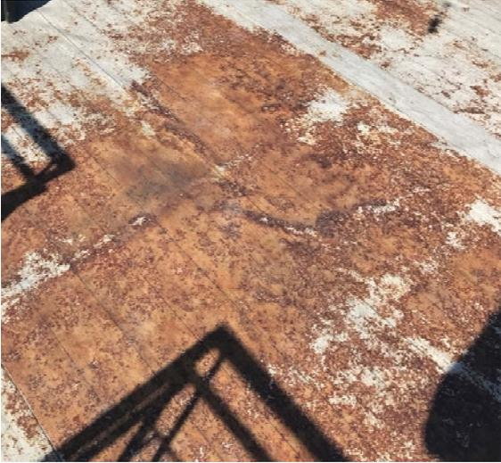
Example 2.) Discoloration of Dec-Tec membrane; cut test revealing OSB as substrate.
